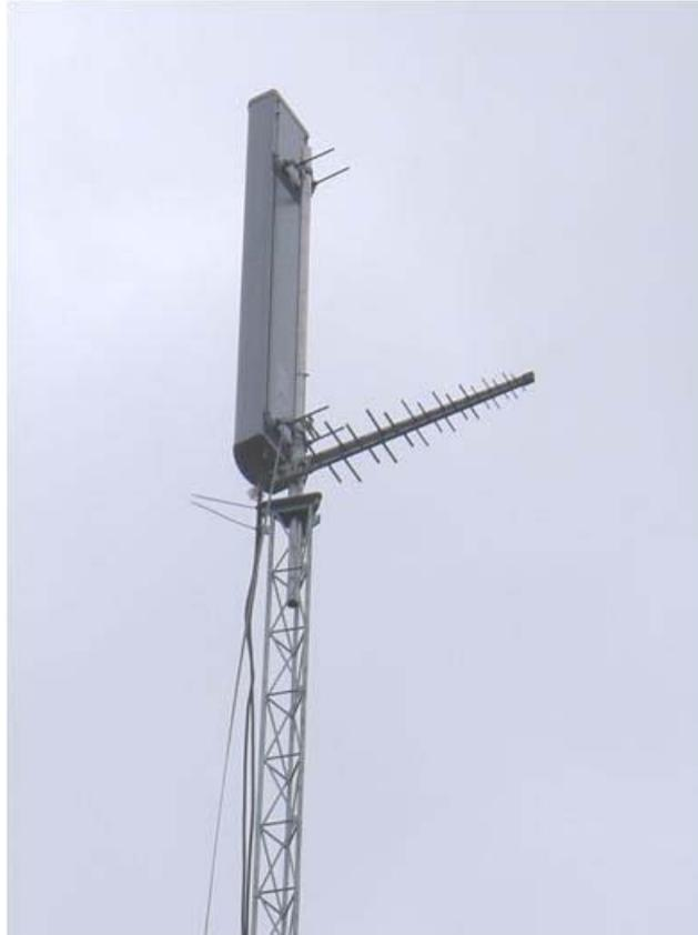
**Figure 7.1: Showing relative location of LTE transmit and DTT receive antennas on trailer mast**
