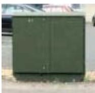
**Street cabinets** are network nodes providing direct or indirect interconnection between the access network and the customer premises, i.e. connect the E-side to the D-side cables of the infrastructure network. In fibre to the cabinet (FTTC) deployments, the role of the street cabinets is crucial, as they terminate the copper network, significantly shortening the copper local loop (referred to as the sub-loop). The street cabinet is also referred to as the primary connection point (PCP).
