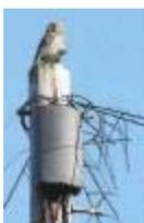
**Distribution points** (DPs) are the last interconnection point in the distribution network before the end customer (forming the start of the last drop). A distribution point is also defined as "*the flexibility point in the distribution network where a multiple tenancy cable is split into single tenancy cables*".<sup>9</sup> An overhead distribution point is recognisable by a small box mounted on a pole; an underground distribution point is typically located in a chamber.
