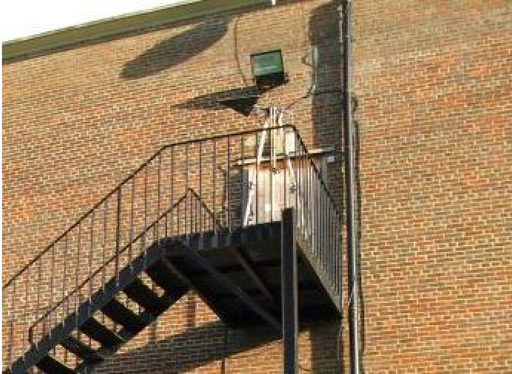
Figure 7: Picture of DVB-T Transmitter
