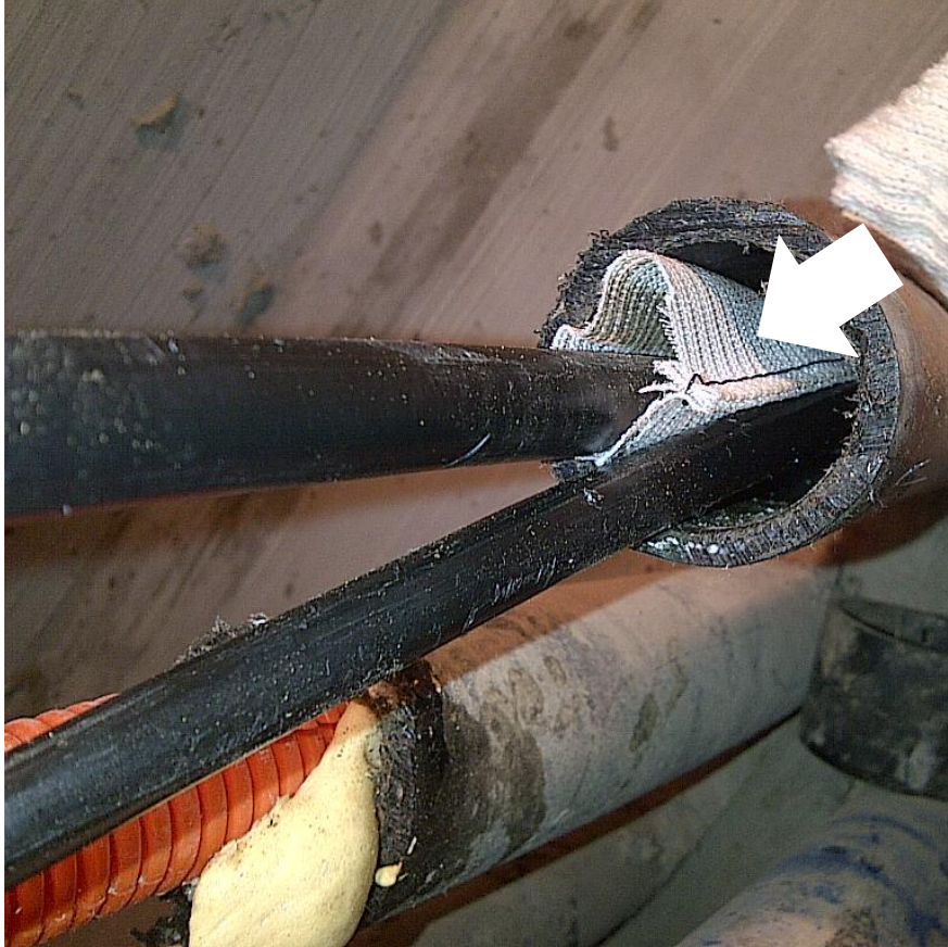
Figure 4.1: A flexible sub-duct (indicated), containing an optical cable, housed in a rigid duct [Source: Maxcell, 2012]
