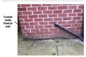
Figure 2.13: 'On-the-ground' duct [Source: Analysys Mason, 2019]
