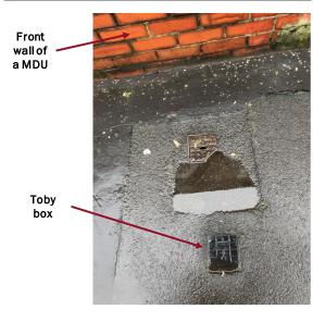
Figure 2.11: Toby box at the edge of a property [Source: Analysys Mason, 2019]
