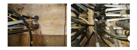
Figure 3.6: Duct nests: close to end user (left) and close to exchange (right) [Source: Analysys Mason]
